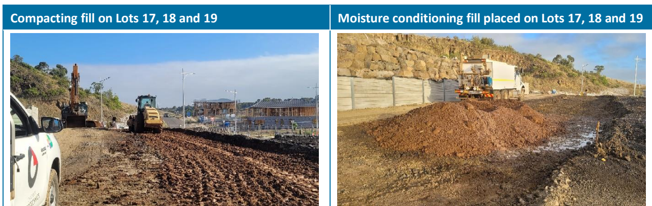
Photographs 4.9 and 4.10: Photographs showing the fill construction on Lots 18 and 19
